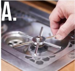
(A) Replace the actuator star over the valve body.
